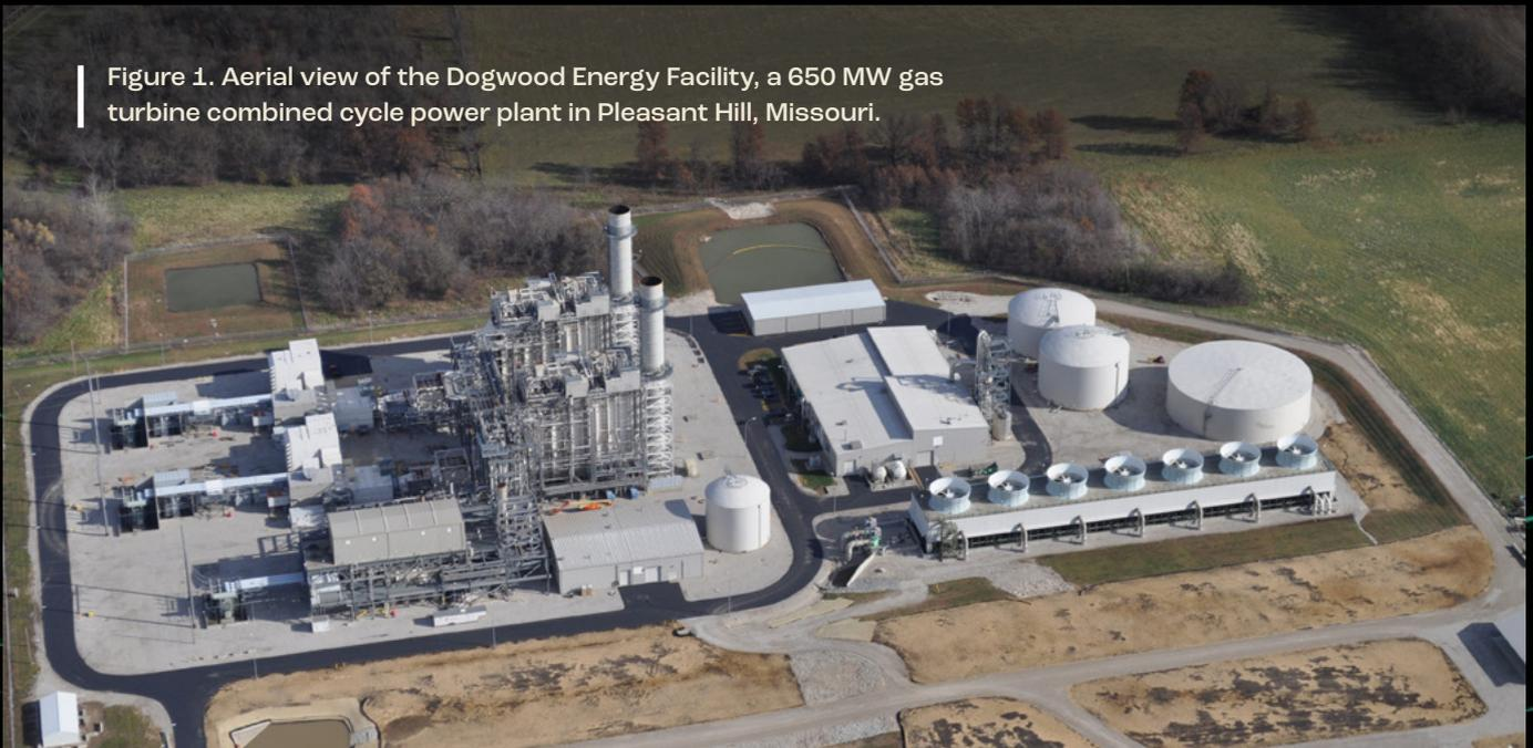
uct. Thus, operating alone, the thermal efficiencies of the Brayton and Rankine cycles can be taken, say, to be about 40 percent and 30 percent respectively. Together in a gas turbine combined cycle plant, they achieve an estimated average 58 percent thermal efficiency, a remarkable increase, and a value greater than either of the component efficiencies.
